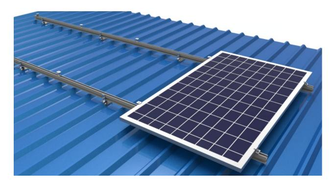
4. Slide the next module against the installed module. Fasten the mid clamps. Install the other modules and clamps this way. Keep modules even.
